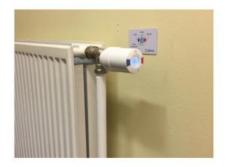
Genius Radiator Valves, replaced existing TRVs
